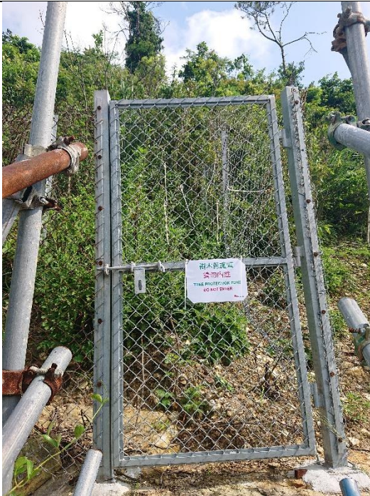
Photo 2 – Current situation of fencing and warning sign
